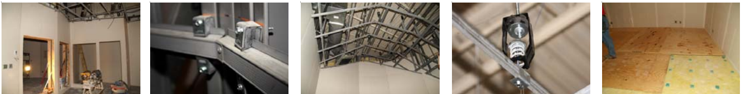
The control room and studio are completely isolated from each other and the rest of the building
