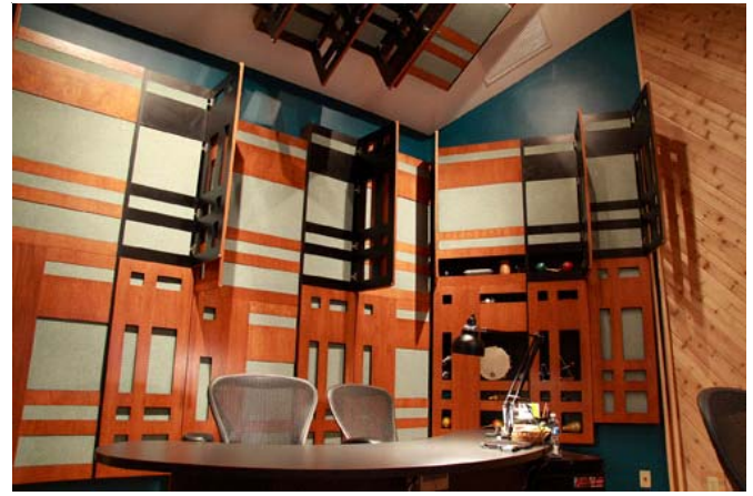
Doors open revealing absorbent fiberglass material
